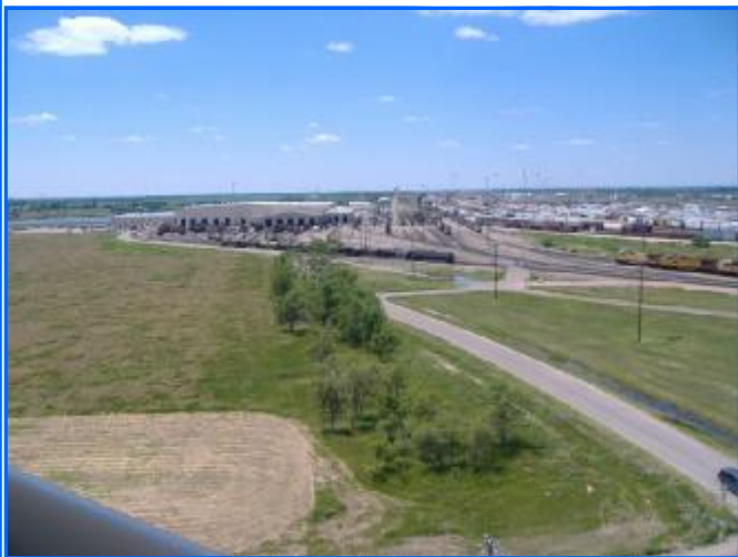
The locomotive shop.
